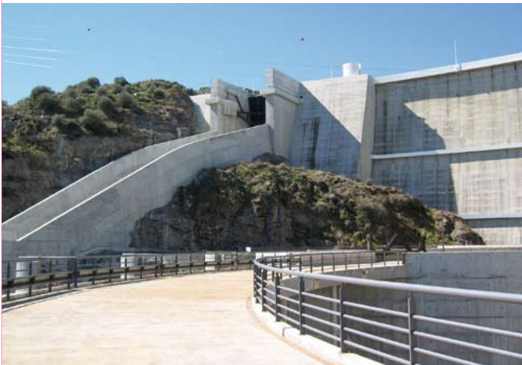
Retention reservoir border Portugal -Spain
