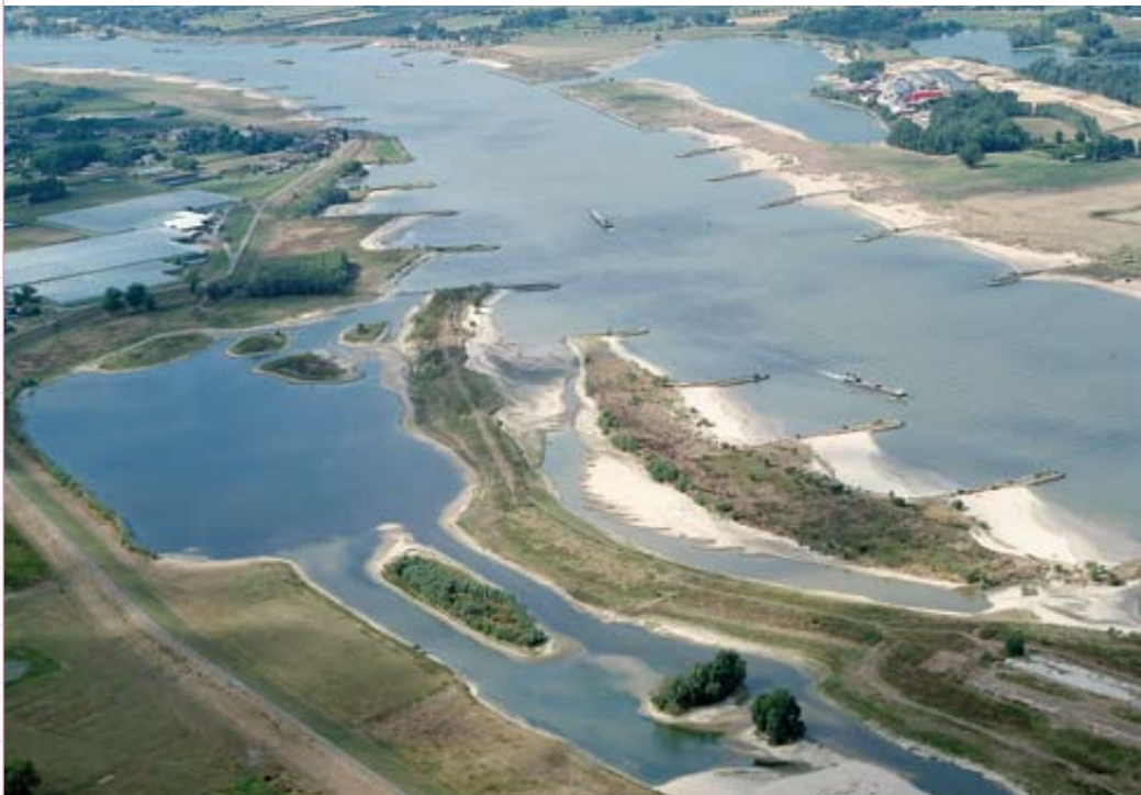
Manmade secondary channels along the river Waal, The Netherlands
