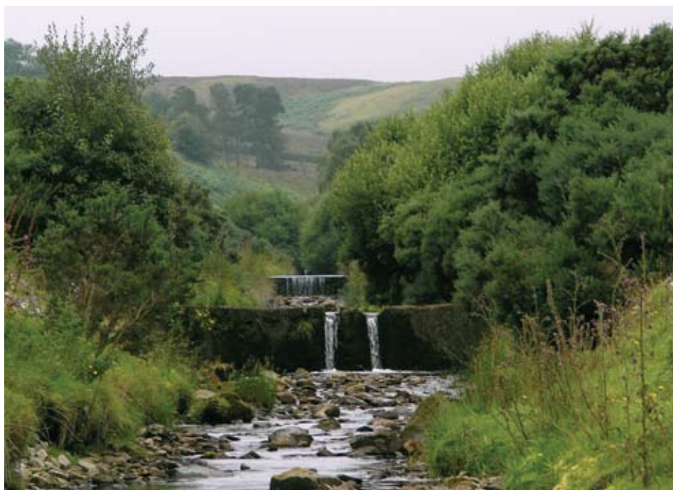
Figure 4 A straight-drop weir, Glensawisk Burn
