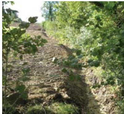
Arterial drainage being dug on Fury
